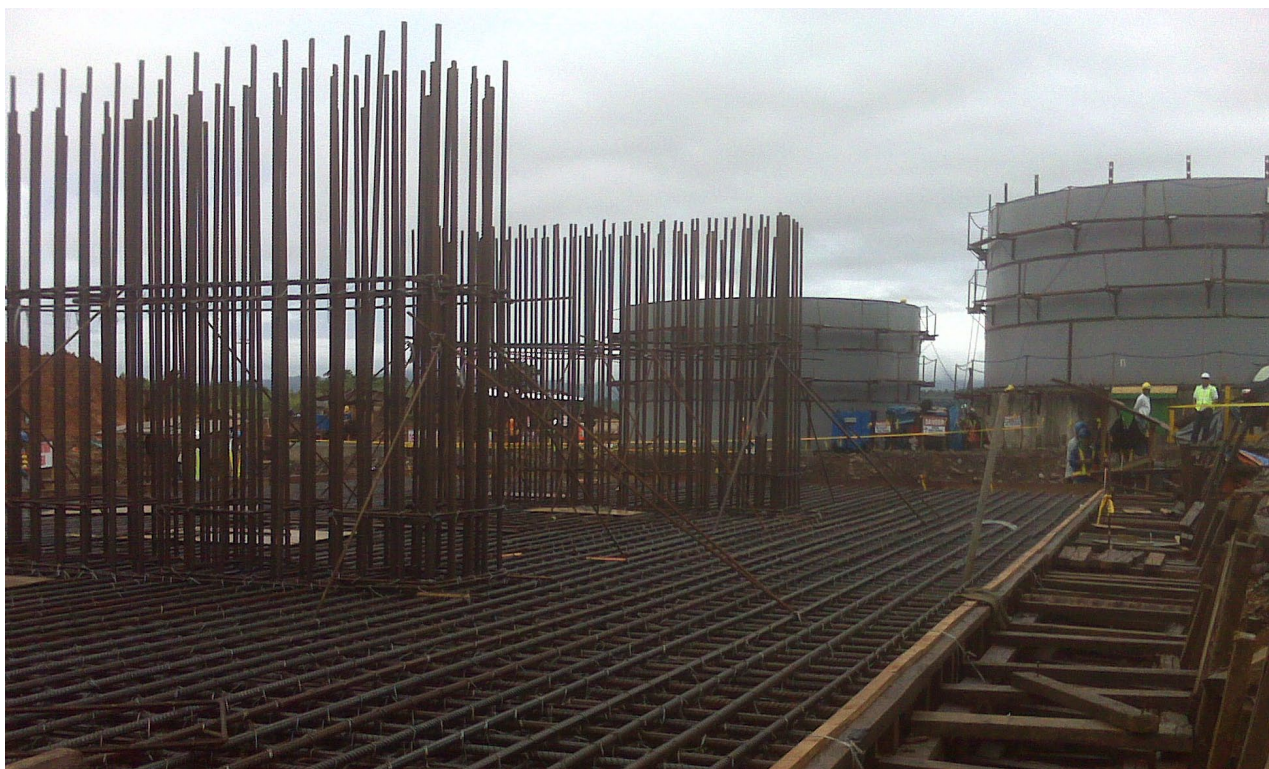
SAG mill foundation formwork and rebar.
