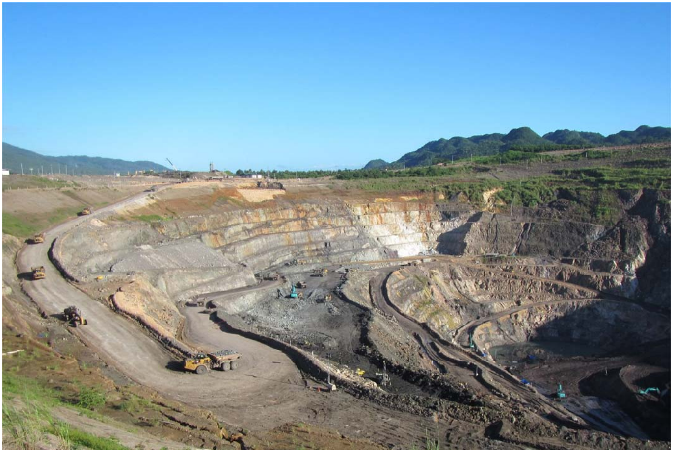
Figure 2: View of the Siana open pit Stage 4 West wall looking north
