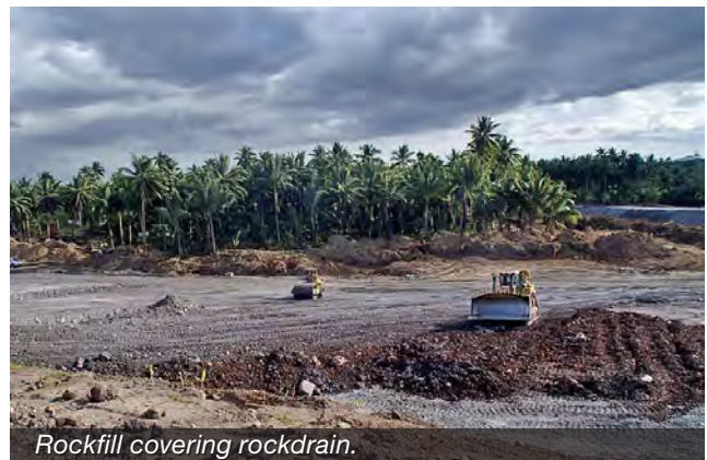
Completed rockfill.
