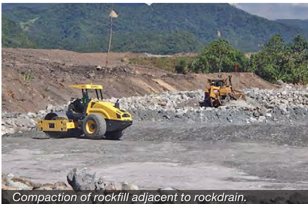
Rockfill covering rockdrain.
