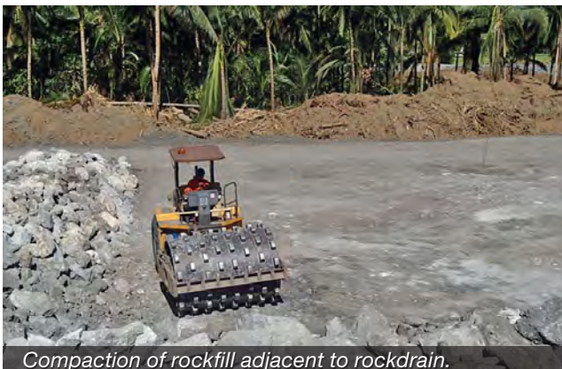
Compaction of rockfill adjacent to rockdrain.
