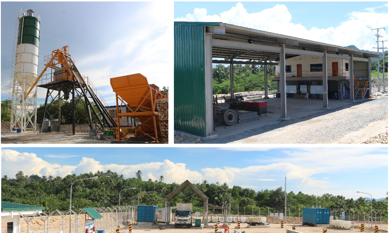
Figures 2, 3 and 4: Underground batching plant (top left), heavy vehicle workshop (top right) and bulk emulsion depot (bottom)
