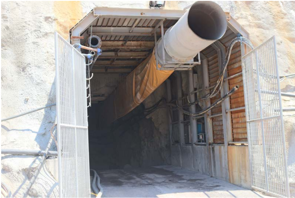
Figure 5: Portal to Main Access Decline
