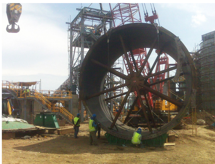
Final preparation prior to SAG mill lift to platform.
