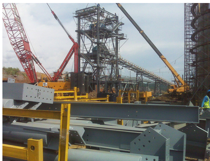
Final steel structure components for cyclone and gravity tower.
