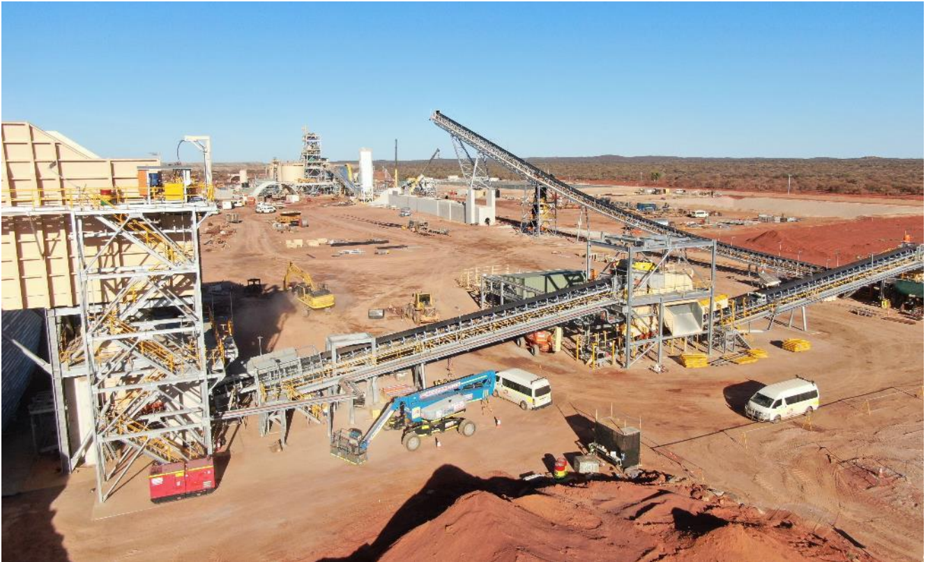
Figure 1: The crushing circuit, with conveyor belts installed and commissioning has commenced.
