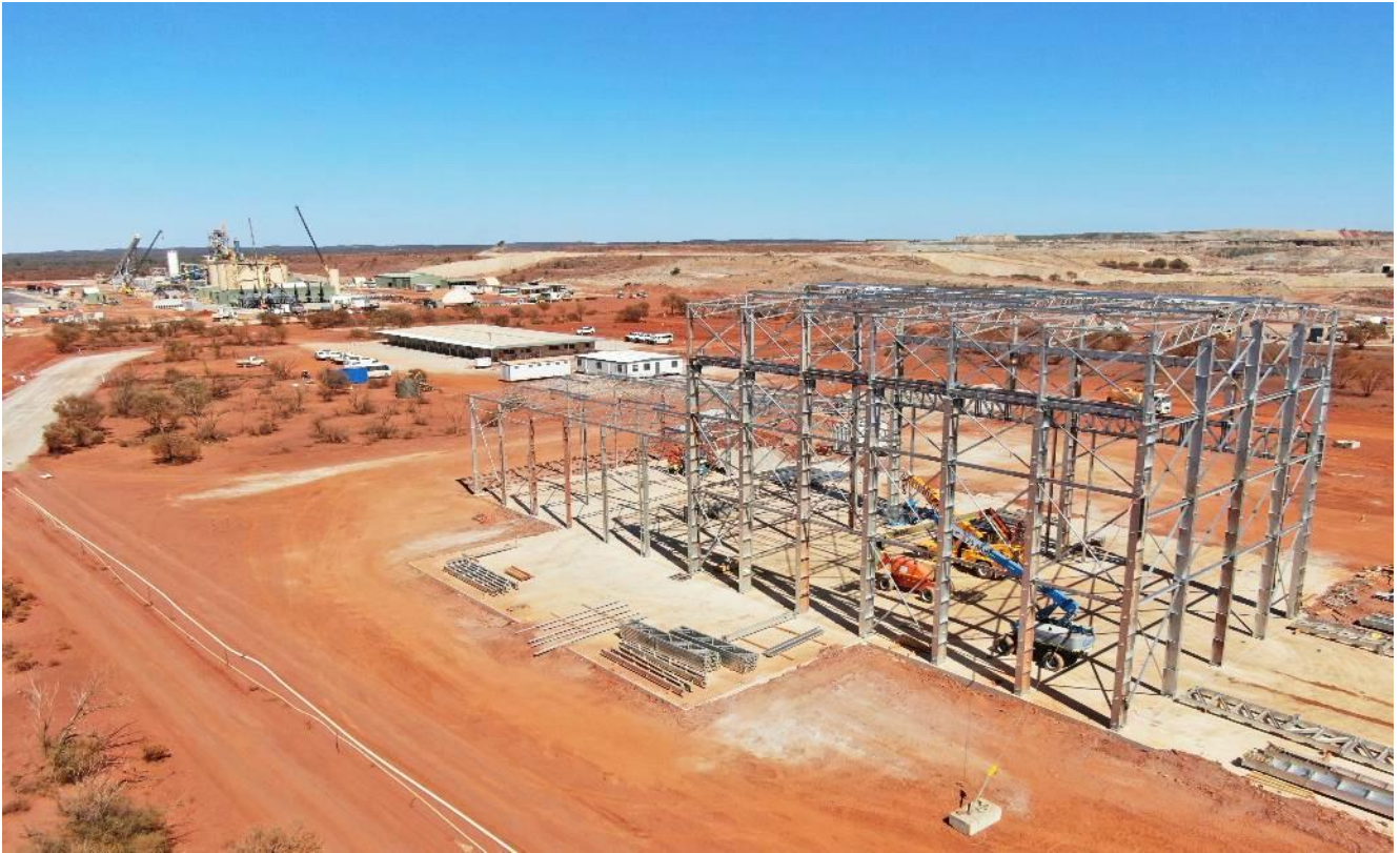
Figure 3: Steel erection for the mine heavy equipment workshop has commenced.
