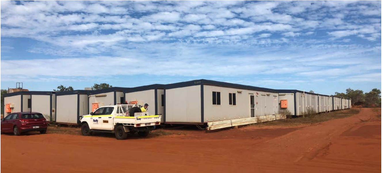
Figure 3. Second-hand portable accommodation units comprising 240 rooms.
