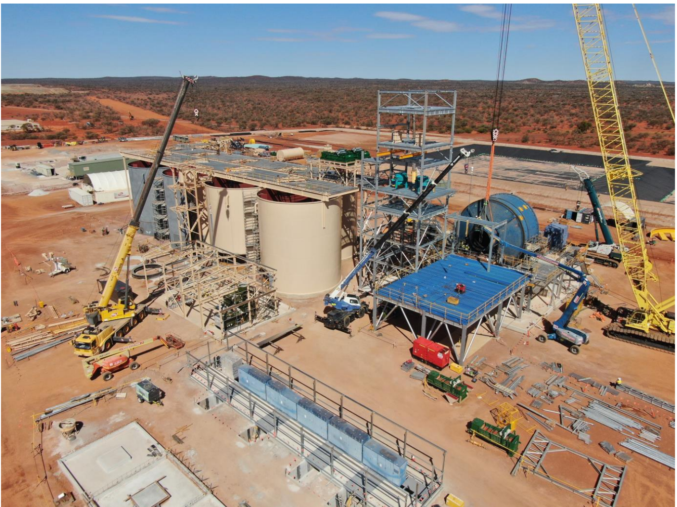
Figure 2: Construction of the KOTH plant as at 15 October 2021.
