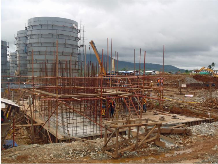
Left: SAG Mill foundation construction shown in the foreground, and CIL tanks in the background.
