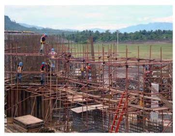
Rebar and formwork preparation for concrete pour of back retaining wall of crusher station.
