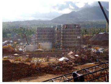
Plant site overview – carbon-in-leach tanks in background, detox tanks middle left and SAG mill foundations near right.
