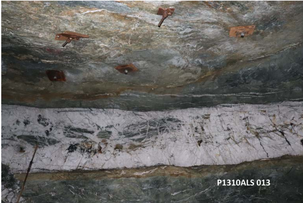
Figure 2: Exposed lode in Pederson 1310 Airleg stope.
