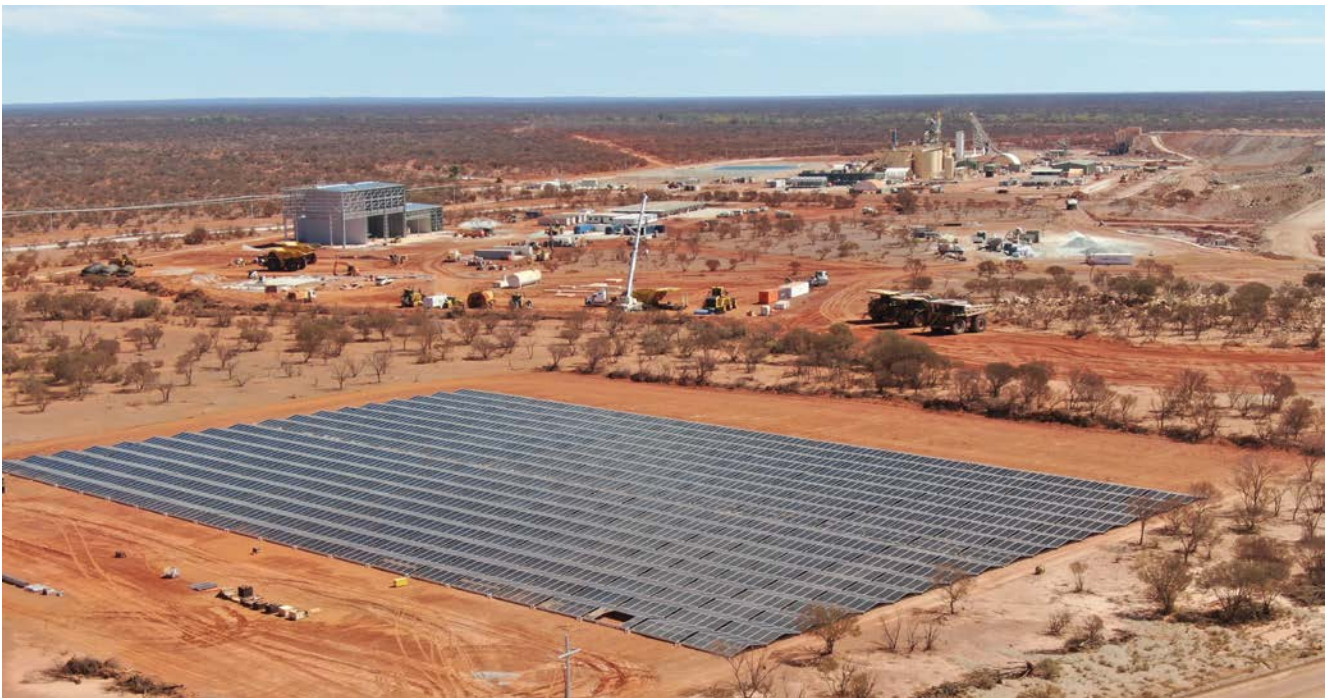
Figure 2: Installation of the solar panel farm is underway.
