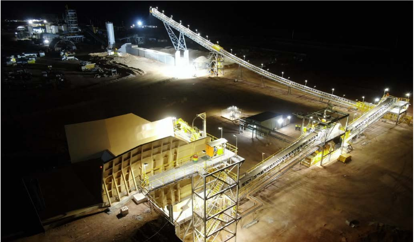
Figure 1: Commissioning of the crushing circuit is nearing completion.
