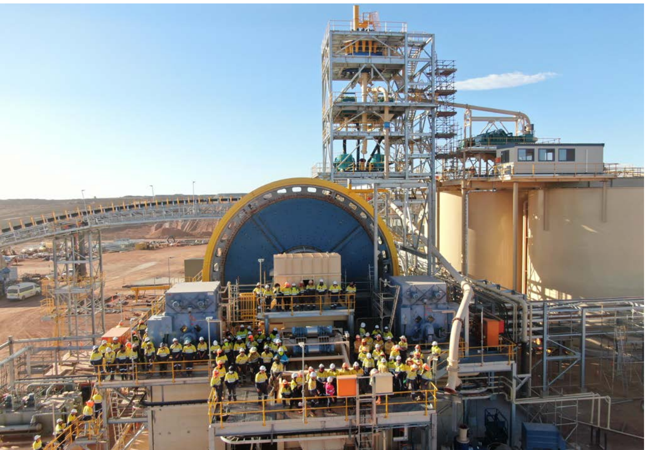
Figure 4: MACA Interquip construction crews in front of the SAG Mill.
