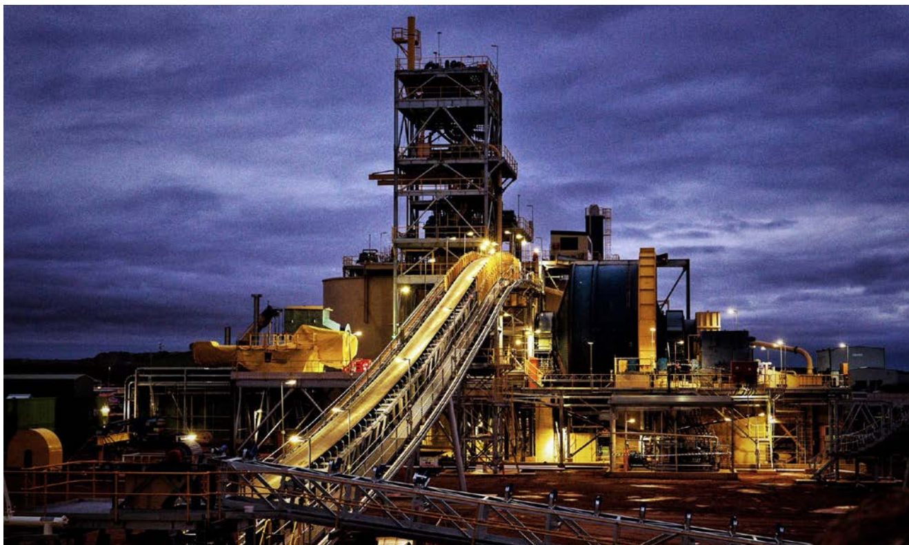
Figure 1: Commissioning of the SAG mill has commenced.
