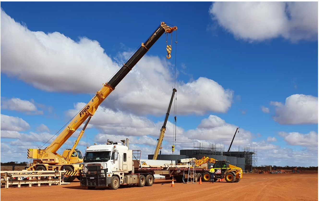
Figure 3: Daily deliveries of structural steel and key equipment are ongoing.
