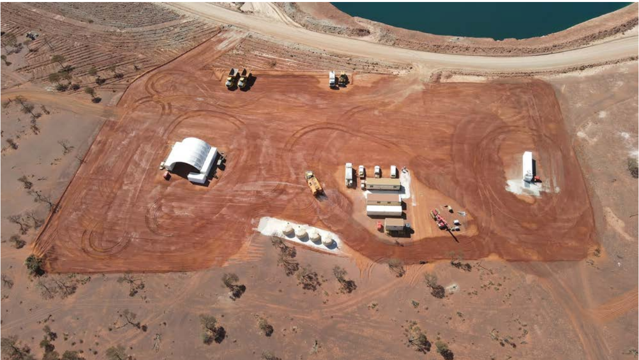
Figure 1: MACA Interquip site establishment.
