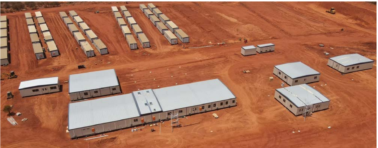
Figure 3: KOTH Village under construction.
