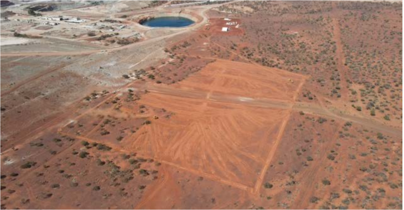
Figure 2: Process facility clearing.
