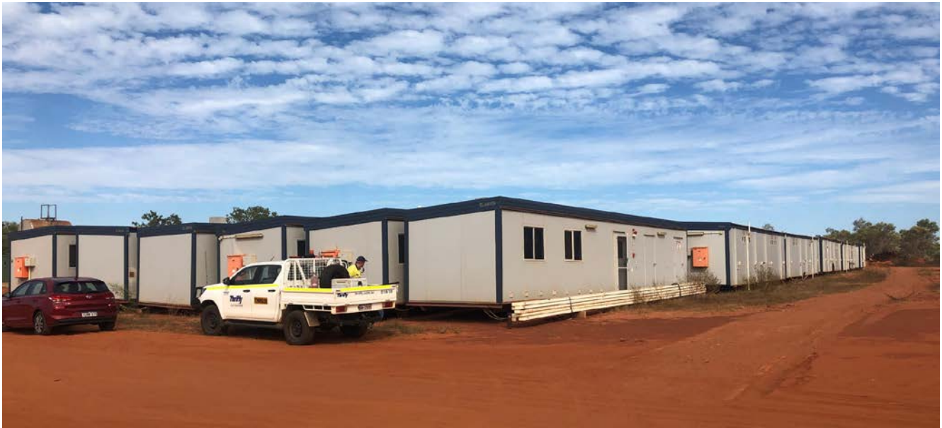
Figure 3. Second-hand portable accommodation units comprising 240 rooms.
