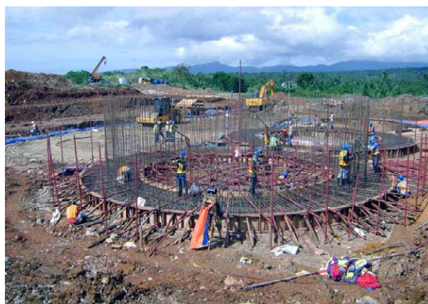
Siana gold mine, carbon in leach tanks foundations.
