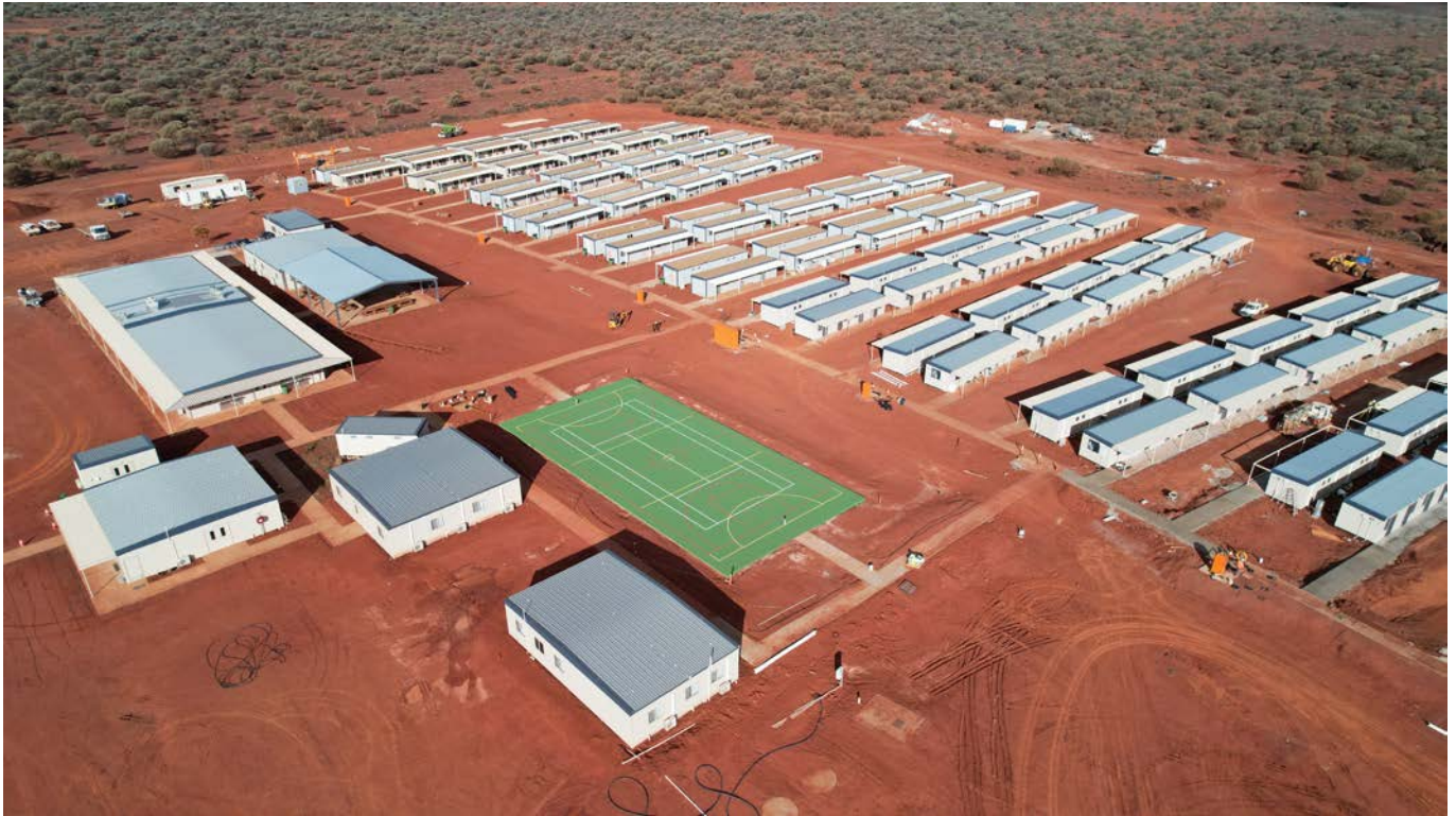
Figure 4: KOTH Village nearing completion.
