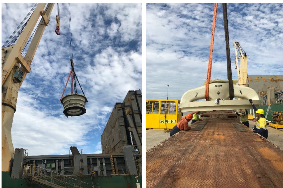
Figure 3: The first of the crusher components have now arrived at Fremantle.
