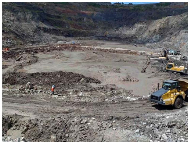
Silt removal from pit (looking south)
