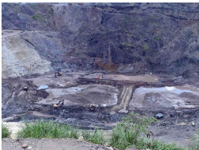
Silt removal from pit (looking east)
