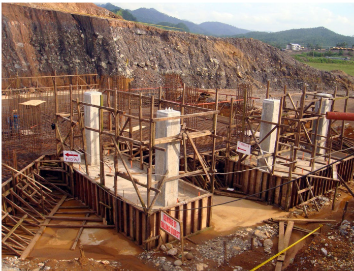
Crusher station ready for major concrete pour.
