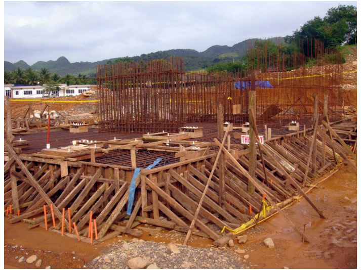
SAG mill formwork with re-bar ready for major concrete pour.
