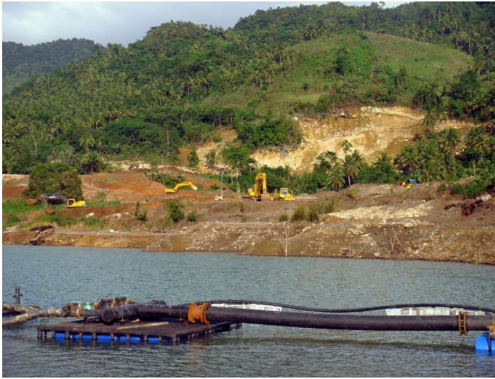
Pit dewatering with cutback activity in background.
