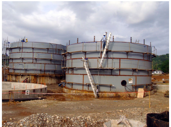
Carbon-in-leach tank erection.
