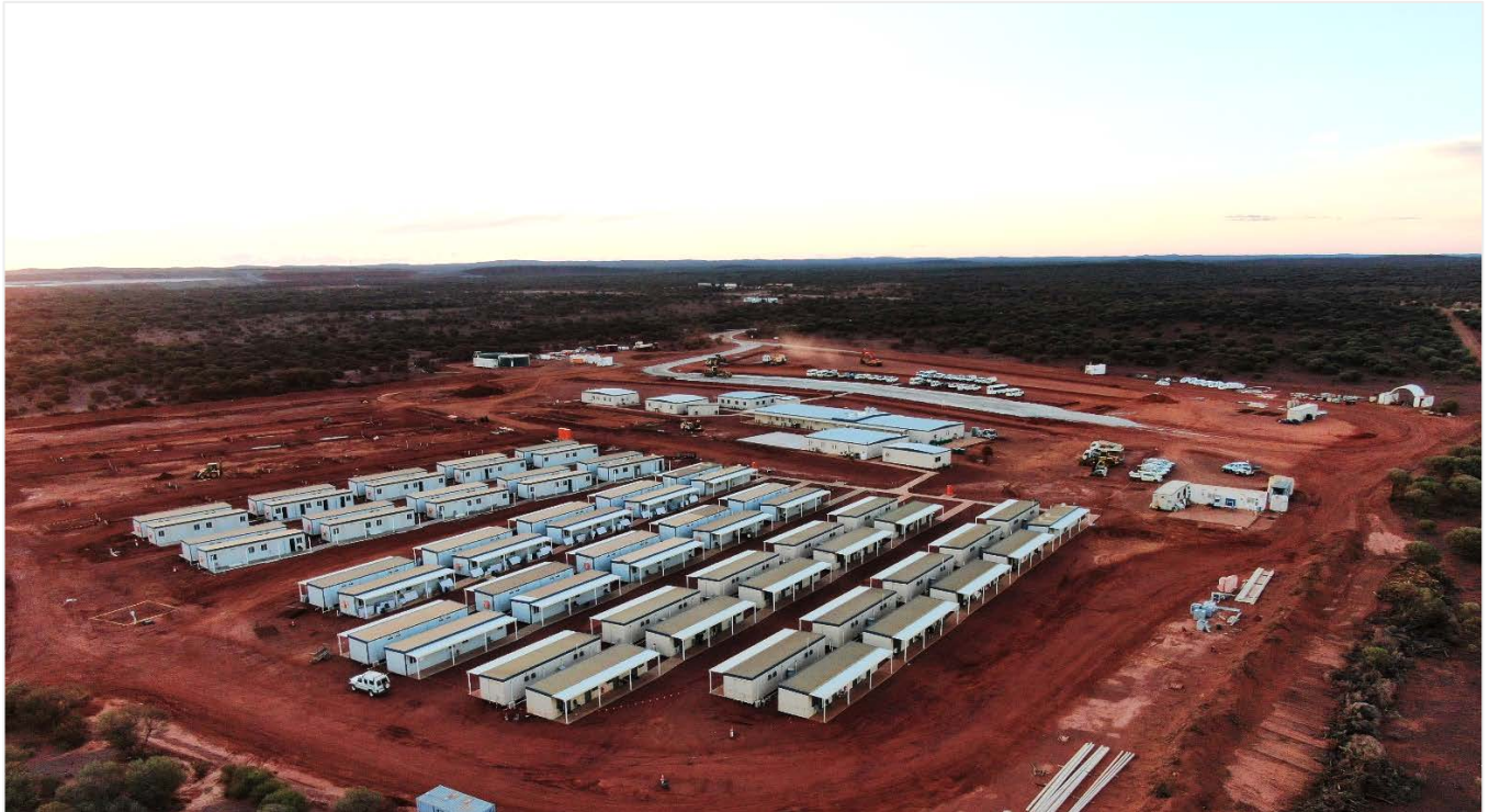
Figure 3: KOTH Village under construction.
