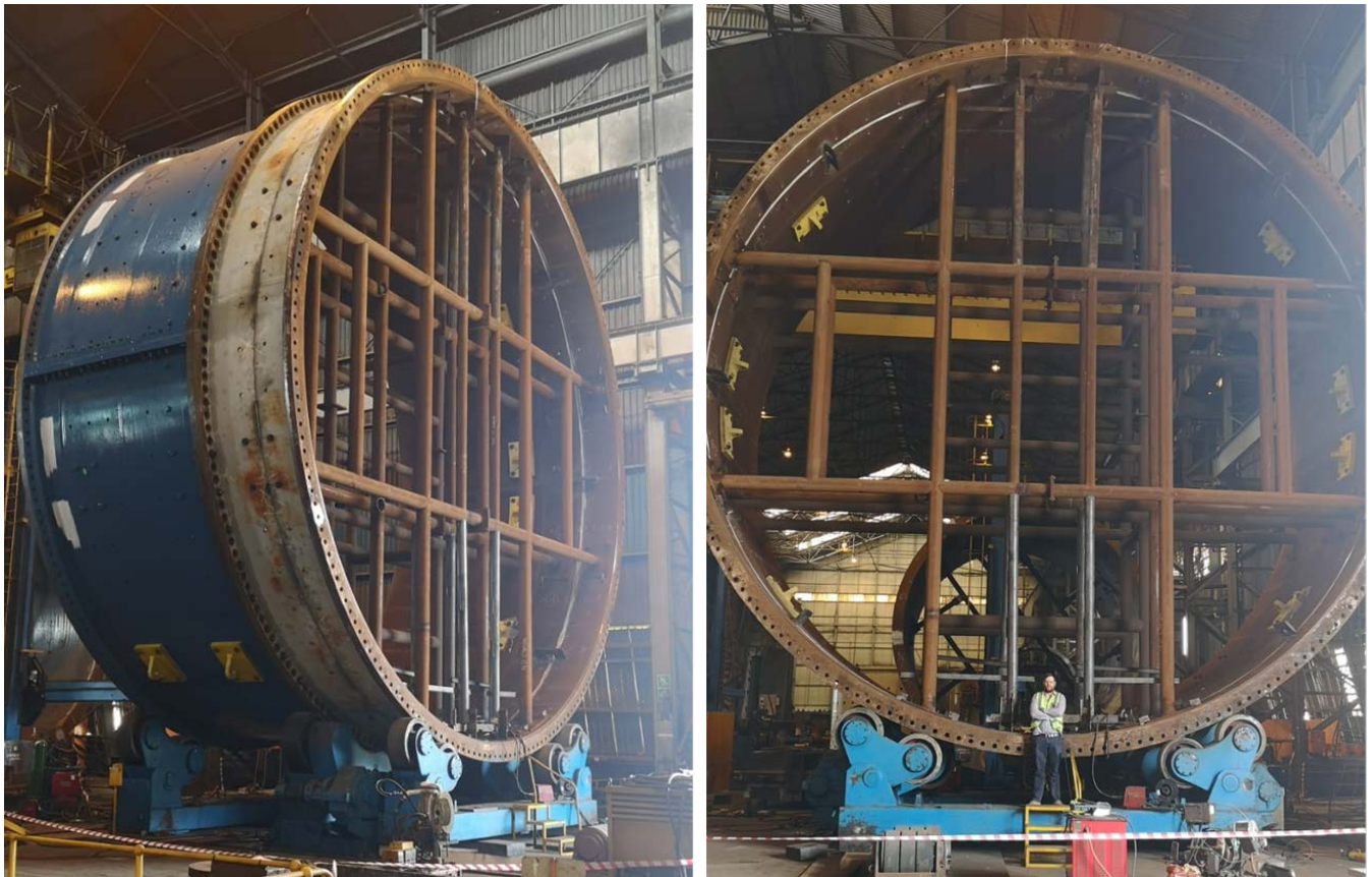
Figure 4: SAG mill shell undergoing refurbishment.
