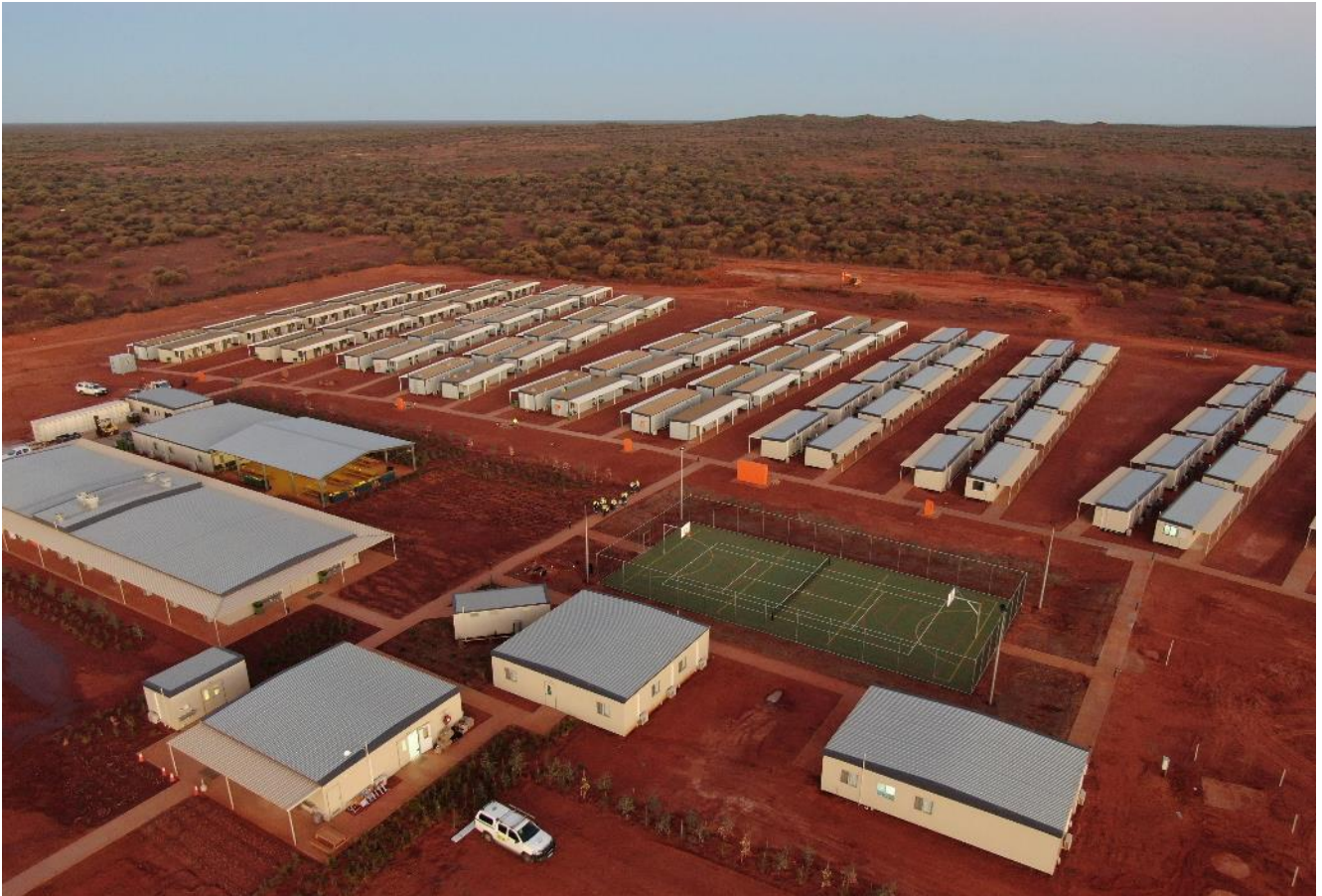
Figure 4: Drone photo showing the KOTH Village at 7 July 2021, which is now fully operational.
