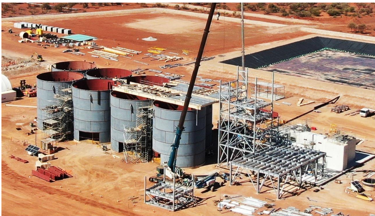
Figure 1: Processing plant and CIL tanks under construction on 7 August 2021.
