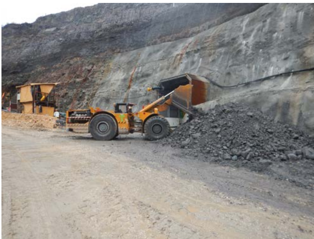
Figures 1 and 2: Portal construction at the Siana Underground Mine
