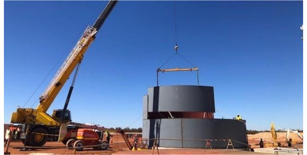
Installation of CIL tanks
