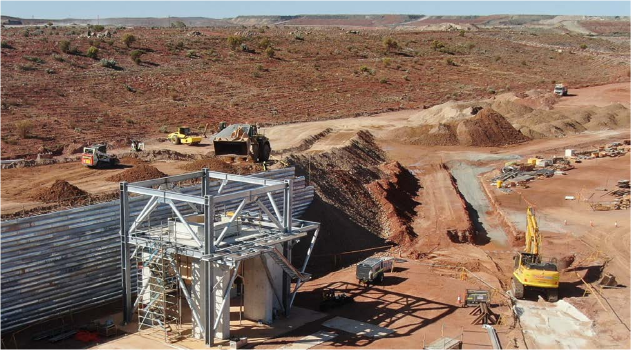
Figure 2: Crusher steelwork being erected and construction of ROM wall underway.
