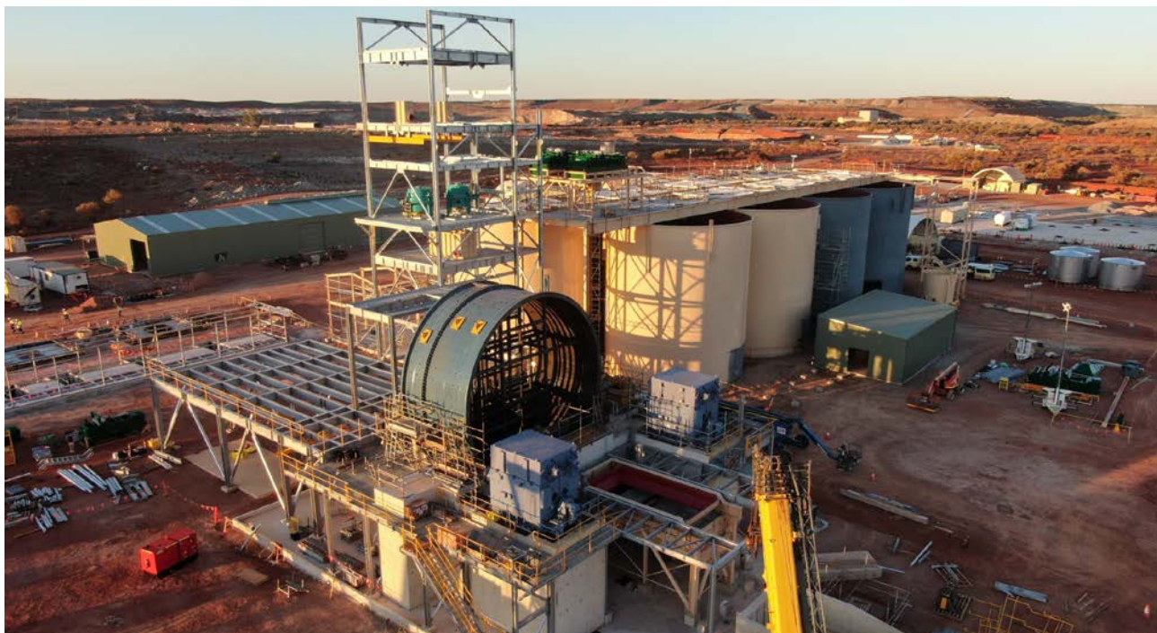
Figure 1: SAG mill motors in position and mill shell currently being assembled.
