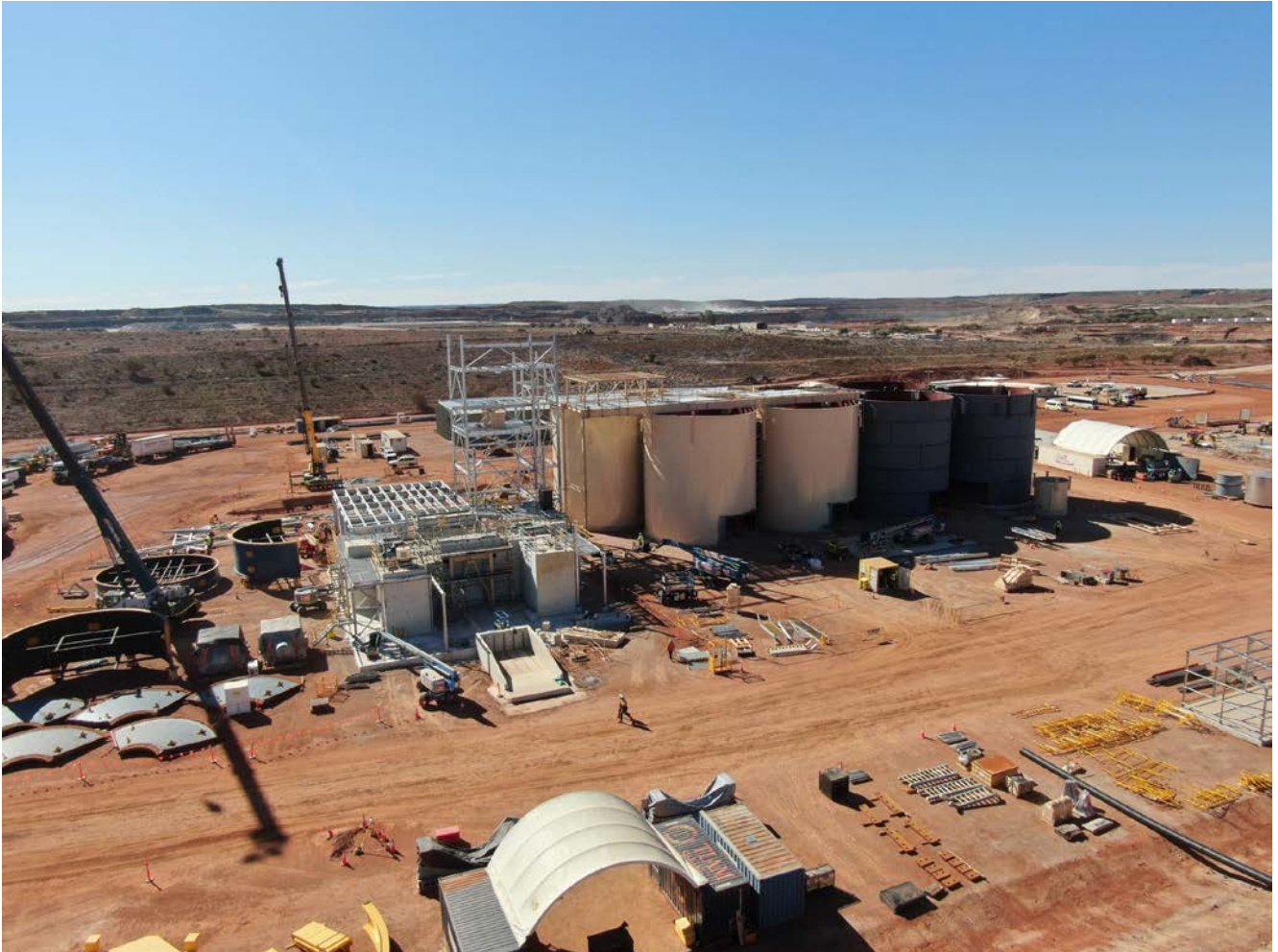
Figure 2: Processing plant and CIL tanks under construction.
