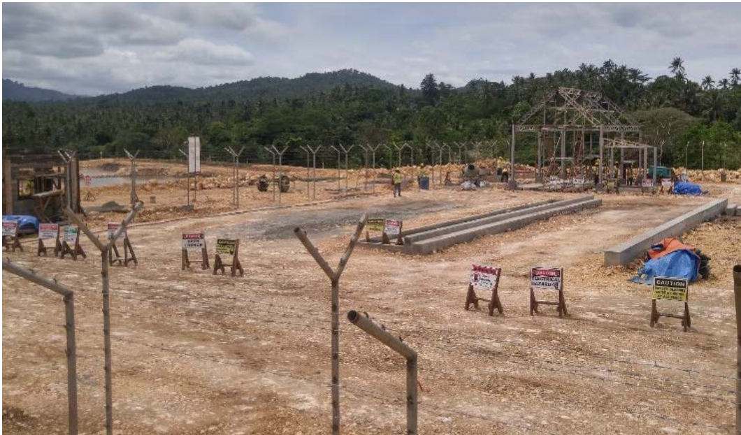
Figure 3: Bulk Emulsion Depot under construction, Siana Gold Project
