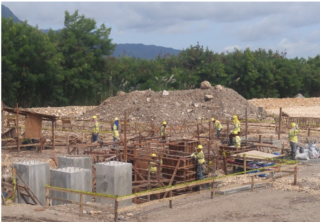
Figure 4: Concrete Batch Plant under construction, Siana Gold Project
